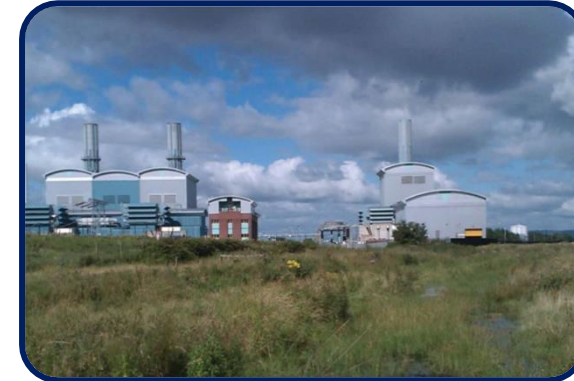
Seabank Power Station
