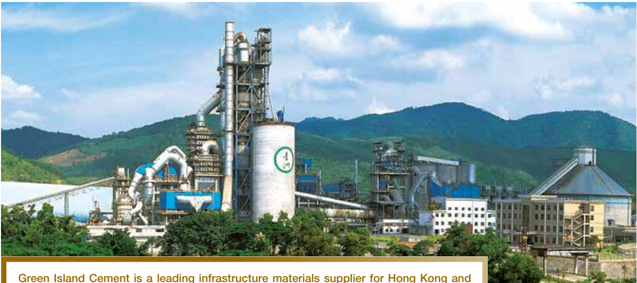
Green Island Cement is a leading infrastructure materials supplier for Hong Kong and the Mainland.
