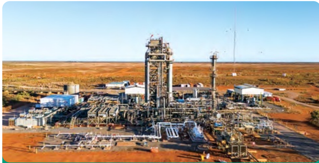
Dampier Bunbury Pipeline's Tubridgi Gas Storage expansion has been completed, allowing for the extraction and sale of additional gas.
