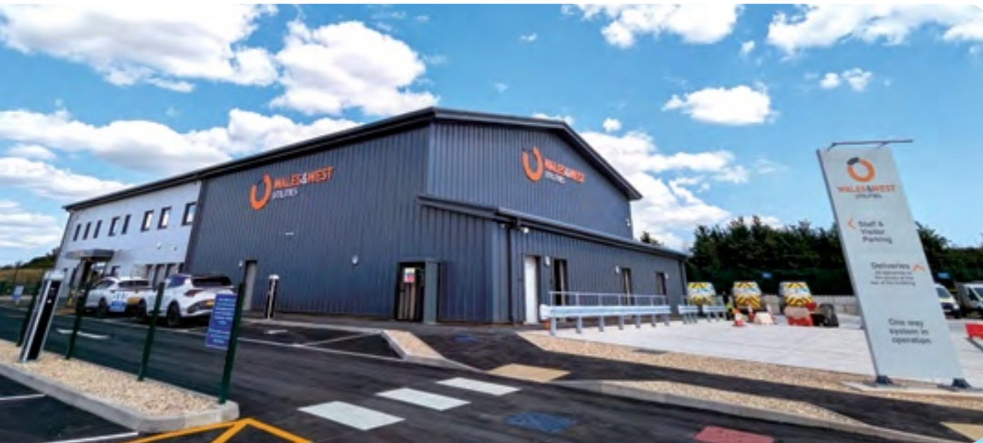
Wales & West Gas Networks received its 12th consecutive Gold Award from RoSPA (Royal Society for the Prevention of Accidents) in recognition of its unwavering dedication to protecting lives and promoting safety while reliably delivering energy.
