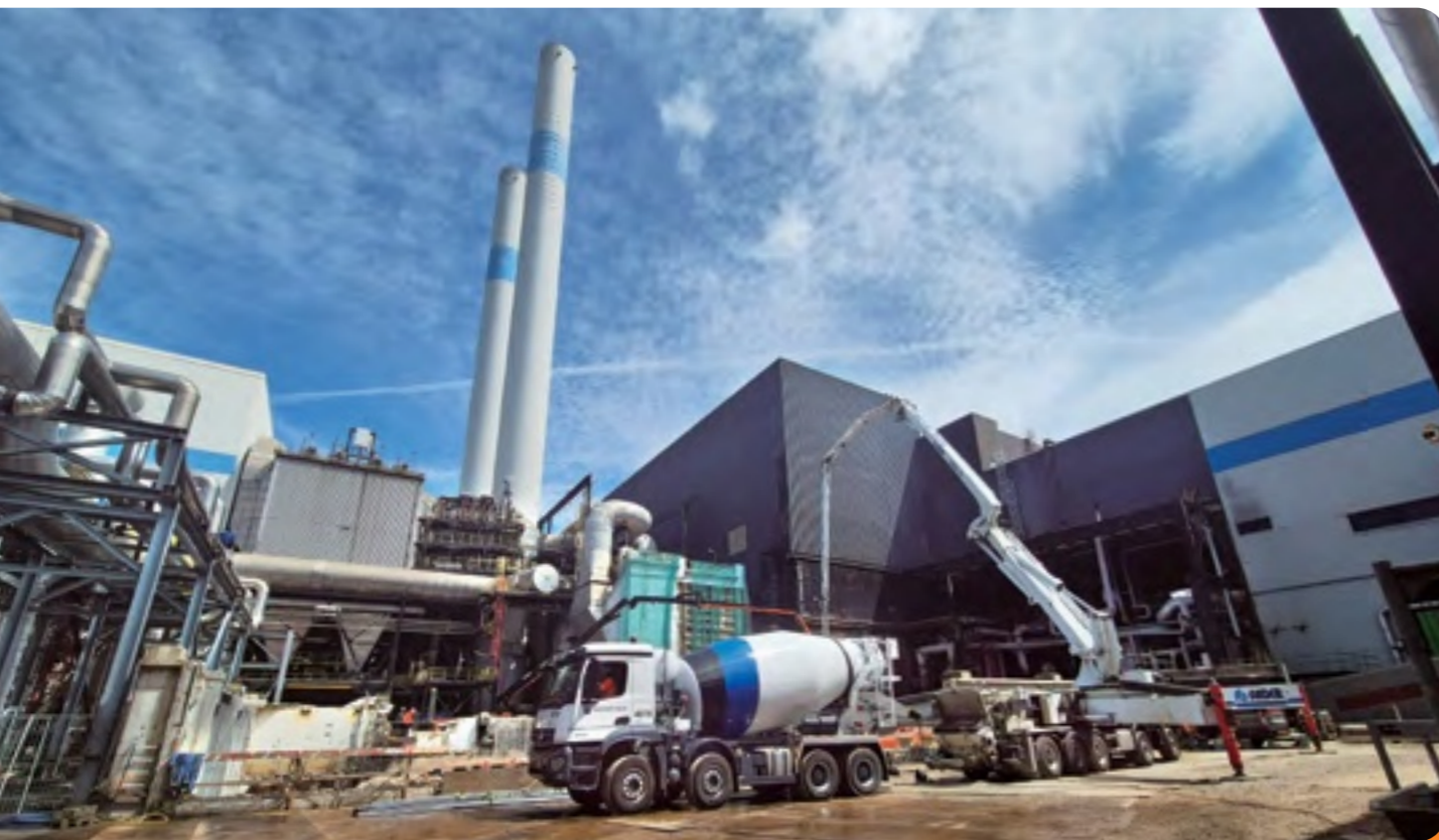
Dutch Enviro Energy's plant in Rozenburg has been in operation for treating waste since March 2025 following the fire in September 2023.
