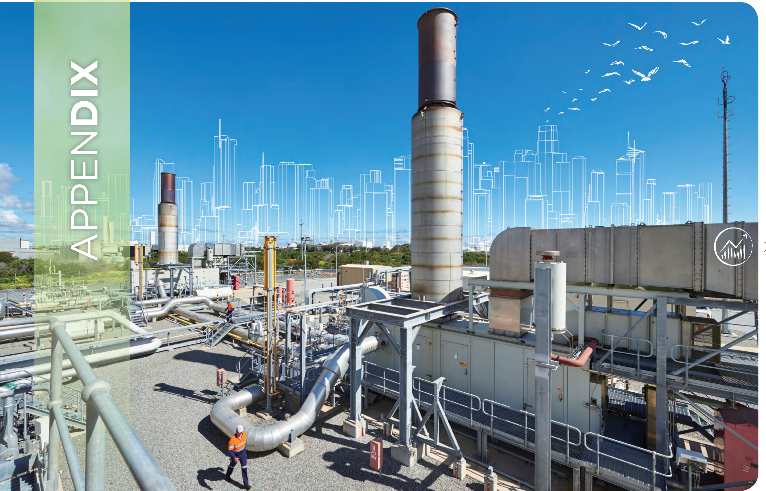
DBP's gas compress station.
