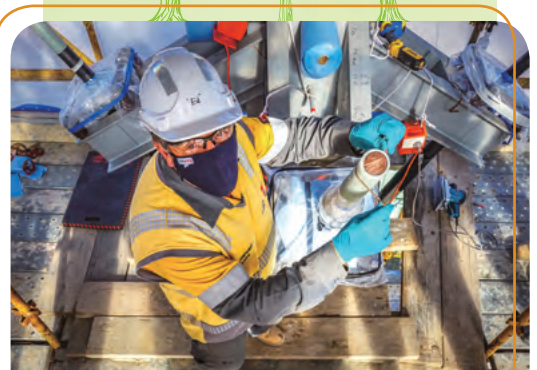
VPNs' field service teams carry out works in full personal protective equipment to keep them safe without compromising reliability.
