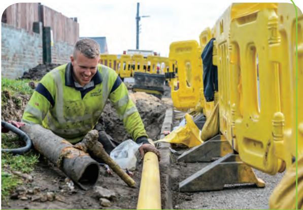
NGN's gas engineer replaced ageing metal pipe with modern equivalents in Sunderland, the UK.
