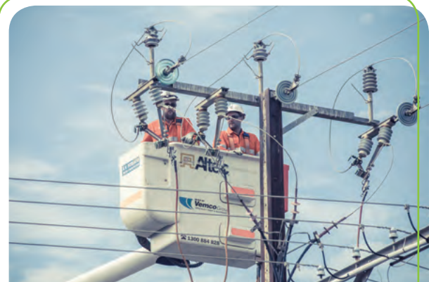
SA Power Networks' technicians carried out work on overhead power lines to maintain safety standards.
