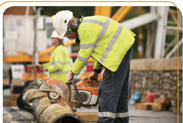
WWU's staff working on Clyst Bridge in Topsham as part of its gas pipe upgrade programme.
