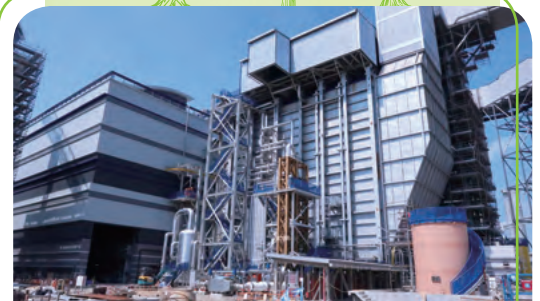
HK Electric's L10 gas-fired combined-cycle generating unit.
