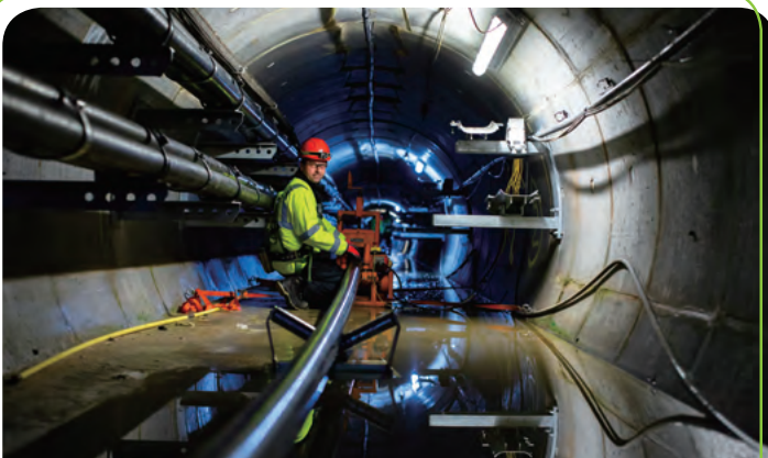
UKPN's engineers install new electricity cables under Battersea in London.
