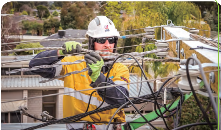
At United Energy, proactive maintenance takes place routinely to ensure reliability levels.
