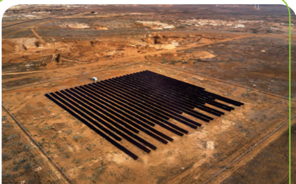
EDL's Coober Pedy Hybrid Renewable power plant.
