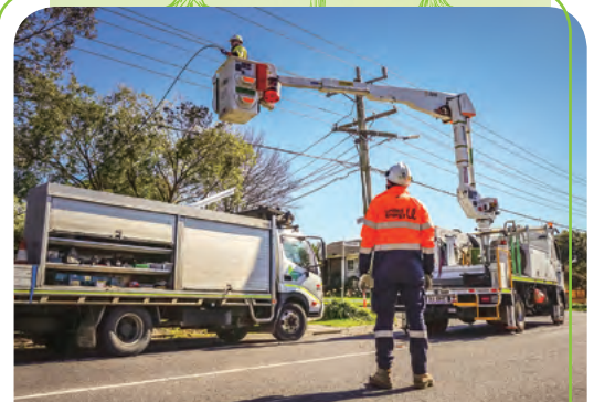
United Energy's workers carried out roadside works. Systematic network maintenance underpins its high reliability levels.
