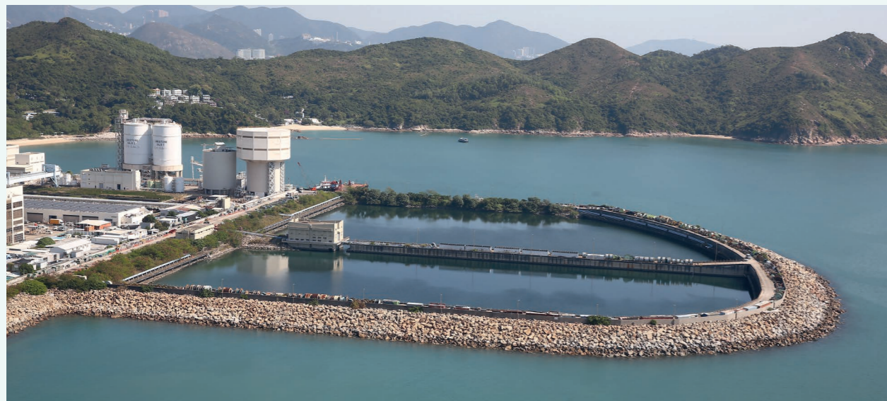
100% of the ash and gypsum produced from HK Electric's Lamma Power Station is reused by third parties for industrial applications. Storage silos and an ash lagoon have been constructed in the Power Station.
