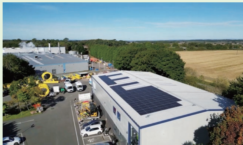
Solar panels at NGN’s depot in Burradon, Newcastle upon Tyne.
