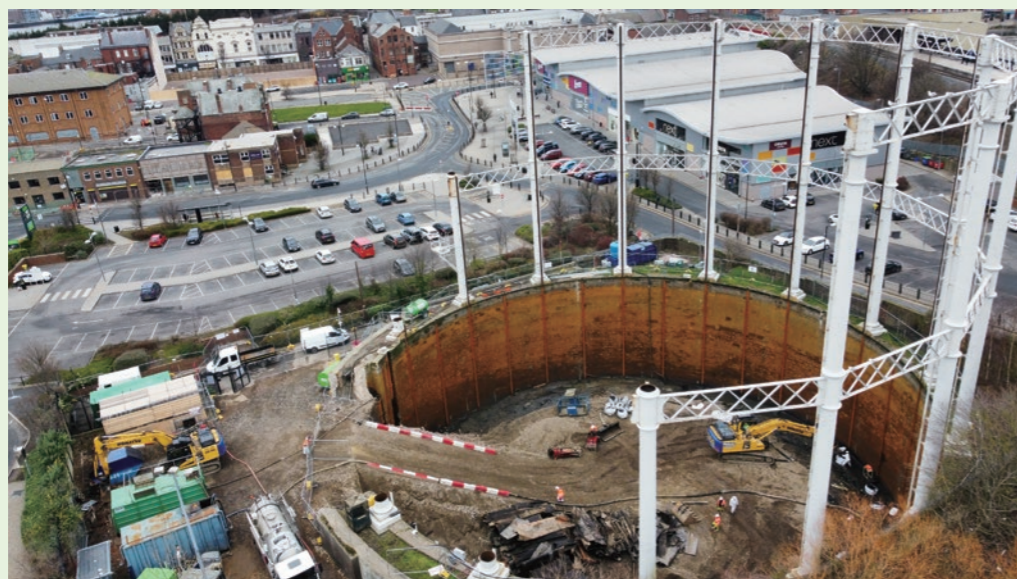
NGN South Shields Gas Holder demolition, image courtesy of Erith Ltd.
